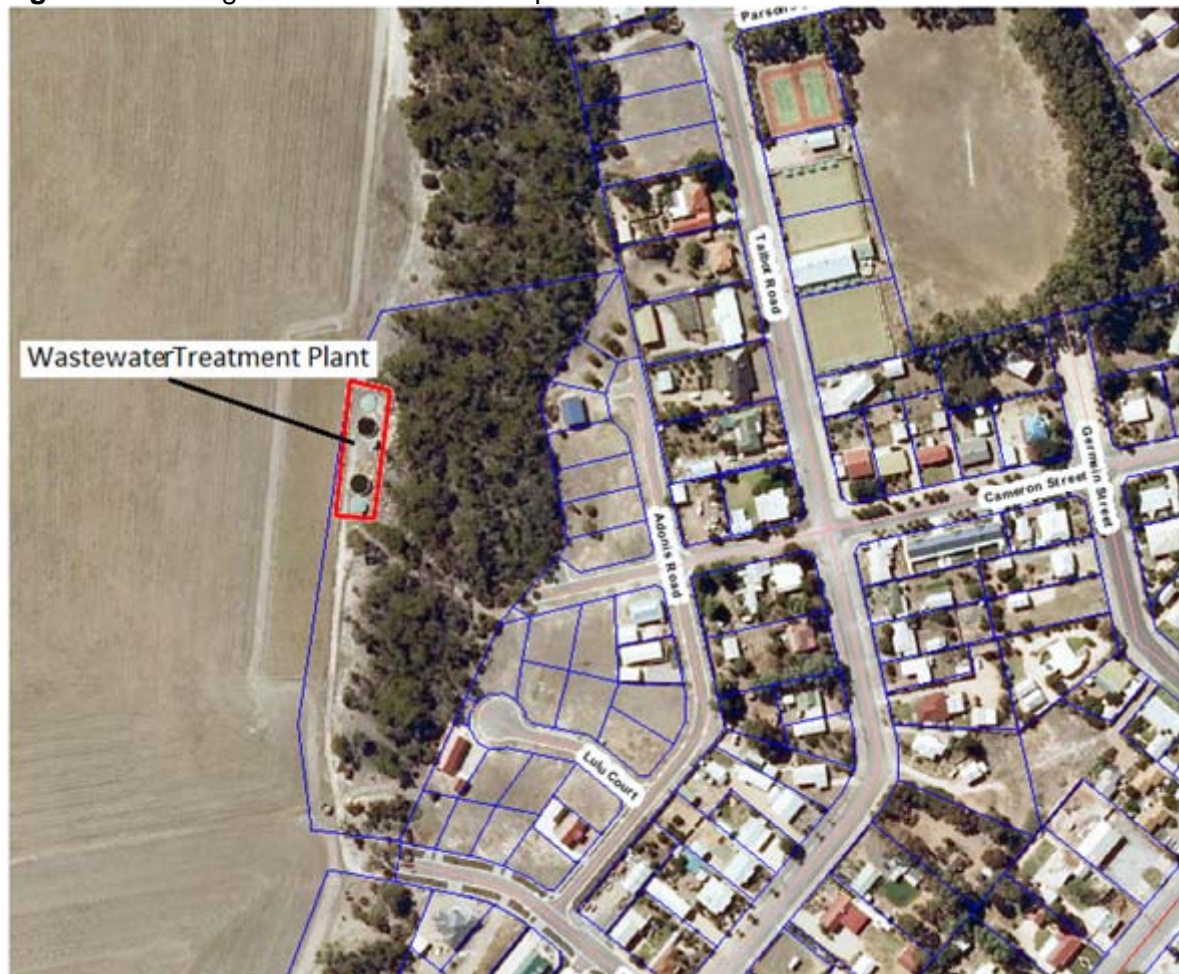
Figure 8: Existing wastewater treatment plant
